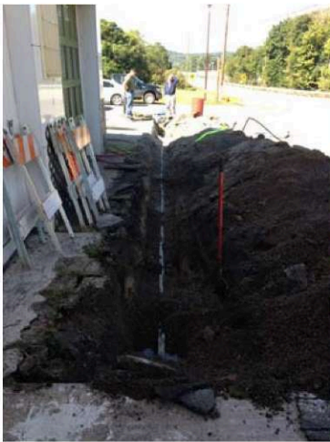
Photos 8,9&10 (9/22/2014): The diesel product line and dispenser area were excavated for visual inspection. Potentially perched water was identified below the product line and dispenser which appeared visibly impacted. However, water sample W-1 was collected at the diesel dispenser, and laboratory analysis reported no detectable COC concentrations. The product line was then completely removed from the ground.
