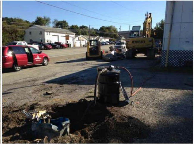
Photos 6&7 (9/22/2014): The diesel dispenser associated with UST #3 was fitted with a plastic drum used as an under dispenser containment sump (UDC). All residual fluids were evacuated from the sump using a drum-top vacuum prior to excavation activities.
