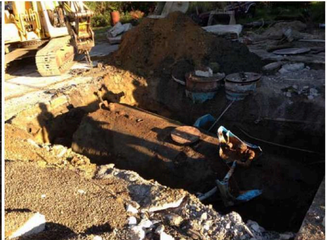
Photos 15&16 (9/23/2014): Concrete paving was removed from over the tanks, and Tank #1 was uncovered. Dark staining was noted on top of the tank near the fill riser and a containment sump which housed vent and vapor recovery piping junctions (left).
