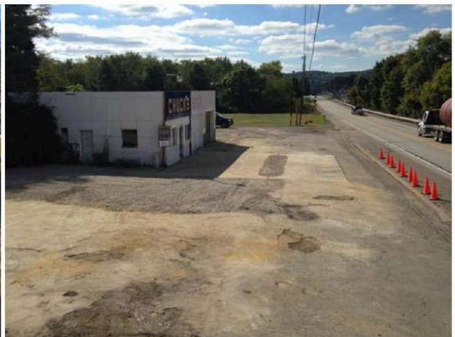
Photos 30&31 (9/24&25/2014): All tanks were verified to be clean and free of hazardous atmospheres then loaded and hauled by Shockey Excavating to Wilson's Scrap Metal in Saltsburg, PA to be recycled. The excavated areas were then backfilled to grade.
