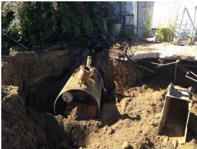
Photos 28&29 (9/24/2014): The Kerosene UST system (UST #007) was found in good condition with no obvious failure points or any signs of contamination.
