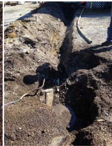
Photos 8,9&10 (9/22/2014): The diesel product line and dispenser area were excavated for visual inspection. Potentially perched water was identified below the product line and dispenser which appeared visibly impacted. However, water sample W-1 was collected at the diesel dispenser, and laboratory analysis reported no detectable COC concentrations. The product line was then completely removed from the ground.
