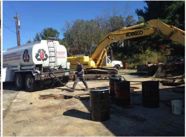
Photos 14&15 (9/23/2014): The drum-top vacuum was used to recover all fluids from tank top sumps, and a pump truck from Environmental Specialists, Inc. was employed to recover a total of 1,075 gallons of residual fluids from the tanks.
