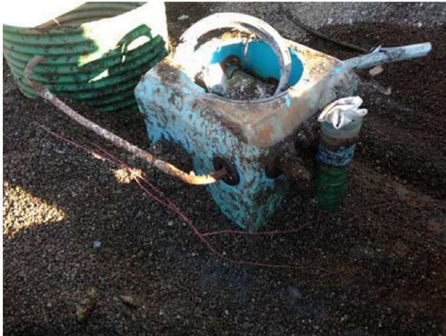
Photos 15&16 (9/23/2014): Concrete paving was removed from over the tanks, and Tank #1 was uncovered. Dark staining was noted on top of the tank near the fill riser and a containment sump which housed vent and vapor recovery piping junctions (left).
