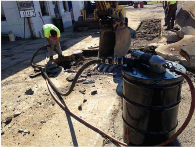
Photos 14&15 (9/23/2014): The drum-top vacuum was used to recover all fluids from tank top sumps, and a pump truck from Environmental Specialists, Inc. was employed to recover a total of 1,075 gallons of residual fluids from the tanks.
