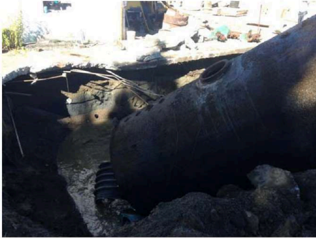
Photos 26&27 (9/24/2014): Showing removal of Tank #3. Dark staining was noted on cavity sidewalls, and water within the cavity carried a light film. Soil samples SW-W and SW-S were collected from these areas of the sidewalls, though field-screening and analytical data suggest that they were not significantly petroleum-impacted. The tank was found in poor condition with deep corrosive pitting, though no obvious holes were observed.
