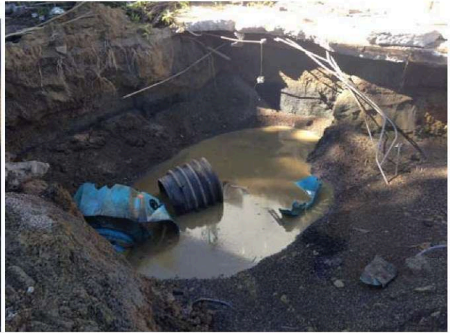
Photos 26&27 (9/24/2014): Showing removal of Tank #3. Dark staining was noted on cavity sidewalls, and water within the cavity carried a light film. Soil samples SW-W and SW-S were collected from these areas of the sidewalls, though field-screening and analytical data suggest that they were not significantly petroleum-impacted. The tank was found in poor condition with deep corrosive pitting, though no obvious holes were observed.
