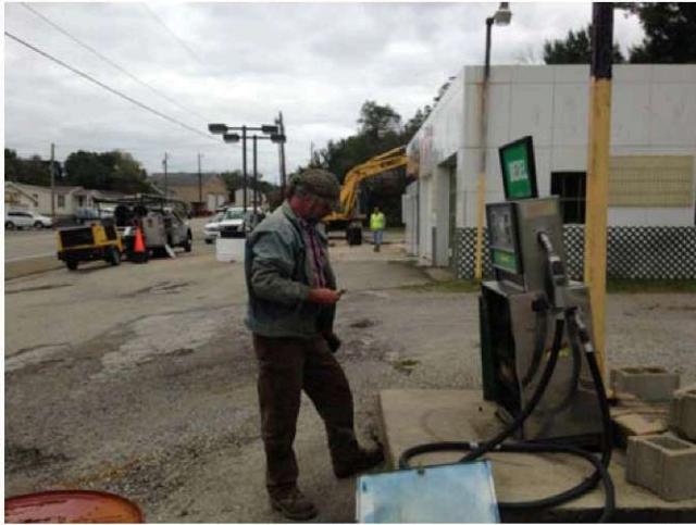
Photos 6&7 (9/22/2014): The diesel dispenser associated with UST #3 was fitted with a plastic drum used as an under dispenser containment sump (UDC). All residual fluids were evacuated from the sump using a drum-top vacuum prior to excavation activities.
