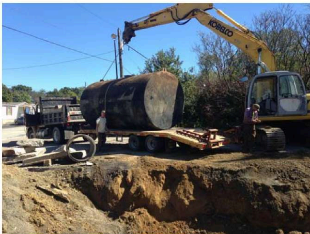
Photos 30&31 (9/24&25/2014): All tanks were verified to be clean and free of hazardous atmospheres then loaded and hauled by Shockey Excavating to Wilson's Scrap Metal in Saltsburg, PA to be recycled. The excavated areas were then backfilled to grade.
