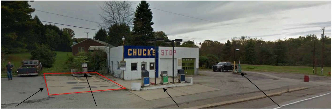
Tank Cavity Kerosene Dispenser Gasoline Dispenser Island Diesel Dispenser Island
