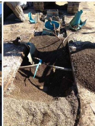
Photos 11,12&13(9/23/2014): The gasoline dispenser island was excavated and product lines were completely removed from the ground by pulling. Potentially perched water below the dispenser island showed no obvious indication of petroleum impact and was sampled as W-2 and W-3 .
