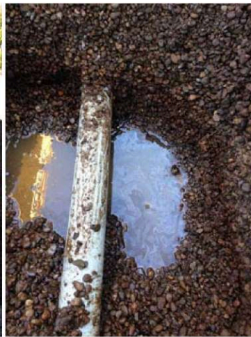
Photos 8,9&10 (9/22/2014): The diesel product line and dispenser area were excavated for visual inspection. Potentially perched water was identified below the product line and dispenser which appeared visibly impacted. However, water sample W-1 was collected at the diesel dispenser, and laboratory analysis reported no detectable COC concentrations. The product line was then completely removed from the ground.
