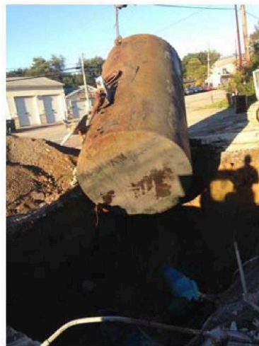
Photos 17&18(9/23/2014): Tank #1 was removed from the cavity. Water in the cavity was observed which exhibited a heavy sheen and produced petroleum odors, and dark staining of the cavity sidewalls was noted. The tank was found in poor condition with deep corrosive pitting, though no obvious holes were observed.
