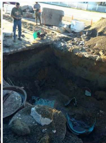
Photos 17&18(9/23/2014): Tank #1 was removed from the cavity. Water in the cavity was observed which exhibited a heavy sheen and produced petroleum odors, and dark staining of the cavity sidewalls was noted. The tank was found in poor condition with deep corrosive pitting, though no obvious holes were observed.
