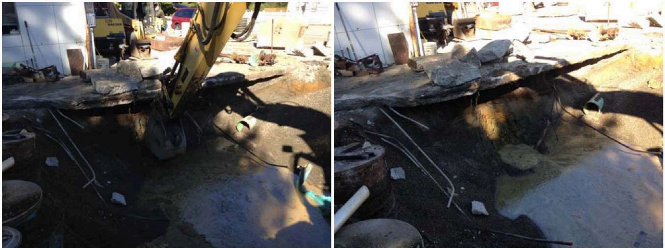
Photos 22&23 (9/24/2014): Showing collection of soil sample SW-W-2 (left) and soil of the sidewall which exhibited no obvious staining.
