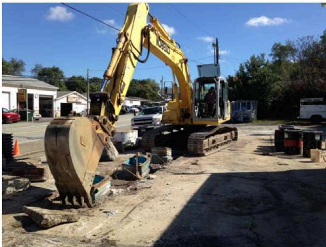
Photos 11,12&13(9/23/2014): The gasoline dispenser island was excavated and product lines were completely removed from the ground by pulling. Potentially perched water below the dispenser island showed no obvious indication of petroleum impact and was sampled as W-2 and W-3 .
