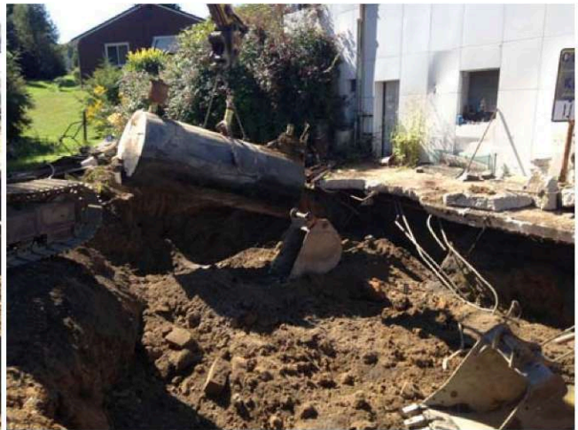
Photos 28&29 (9/24/2014): The Kerosene UST system (UST #007) was found in good condition with no obvious failure points or any signs of contamination.
