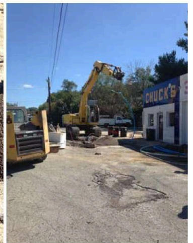
Photos 11,12&13(9/23/2014): The gasoline dispenser island was excavated and product lines were completely removed from the ground by pulling. Potentially perched water below the dispenser island showed no obvious indication of petroleum impact and was sampled as W-2 and W-3 .
