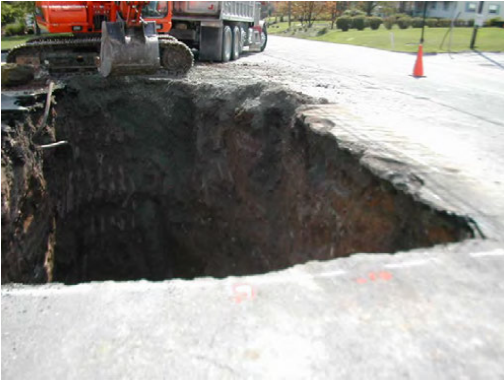
View of Excavation Extent on September 23, 2010 Looking Southeast
