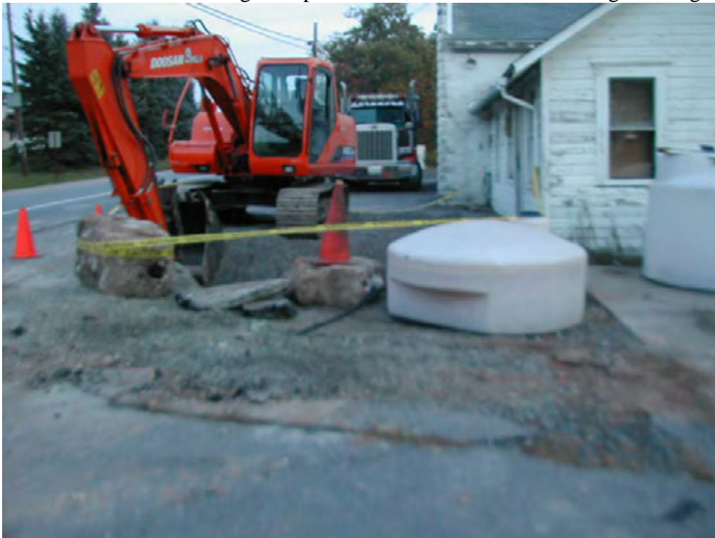
View of Excavation on Morning of September 24, 2010 After Backfilling Looking North
