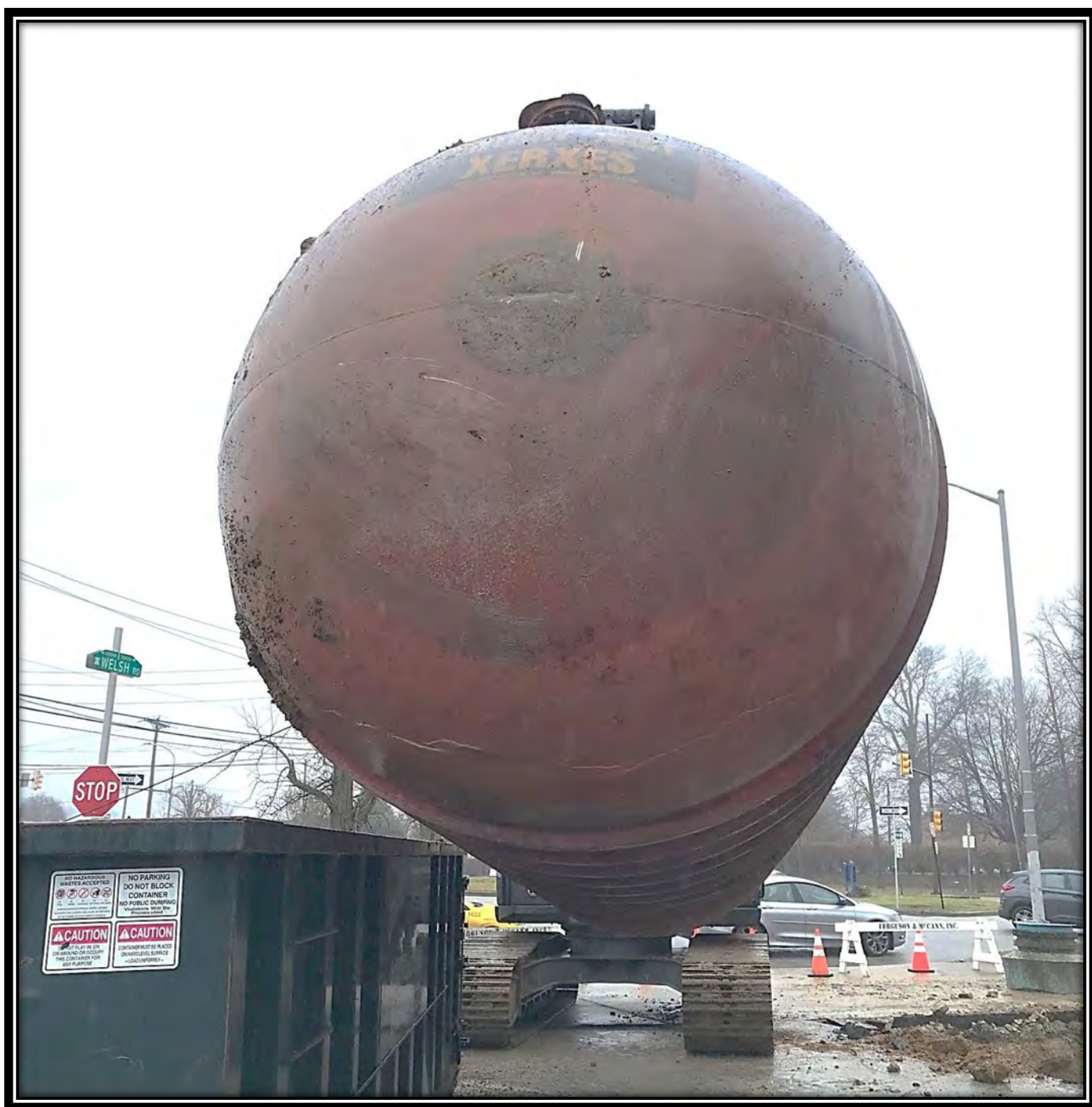
Crack at North End of UST 003. Evidence of a Release Observed.
