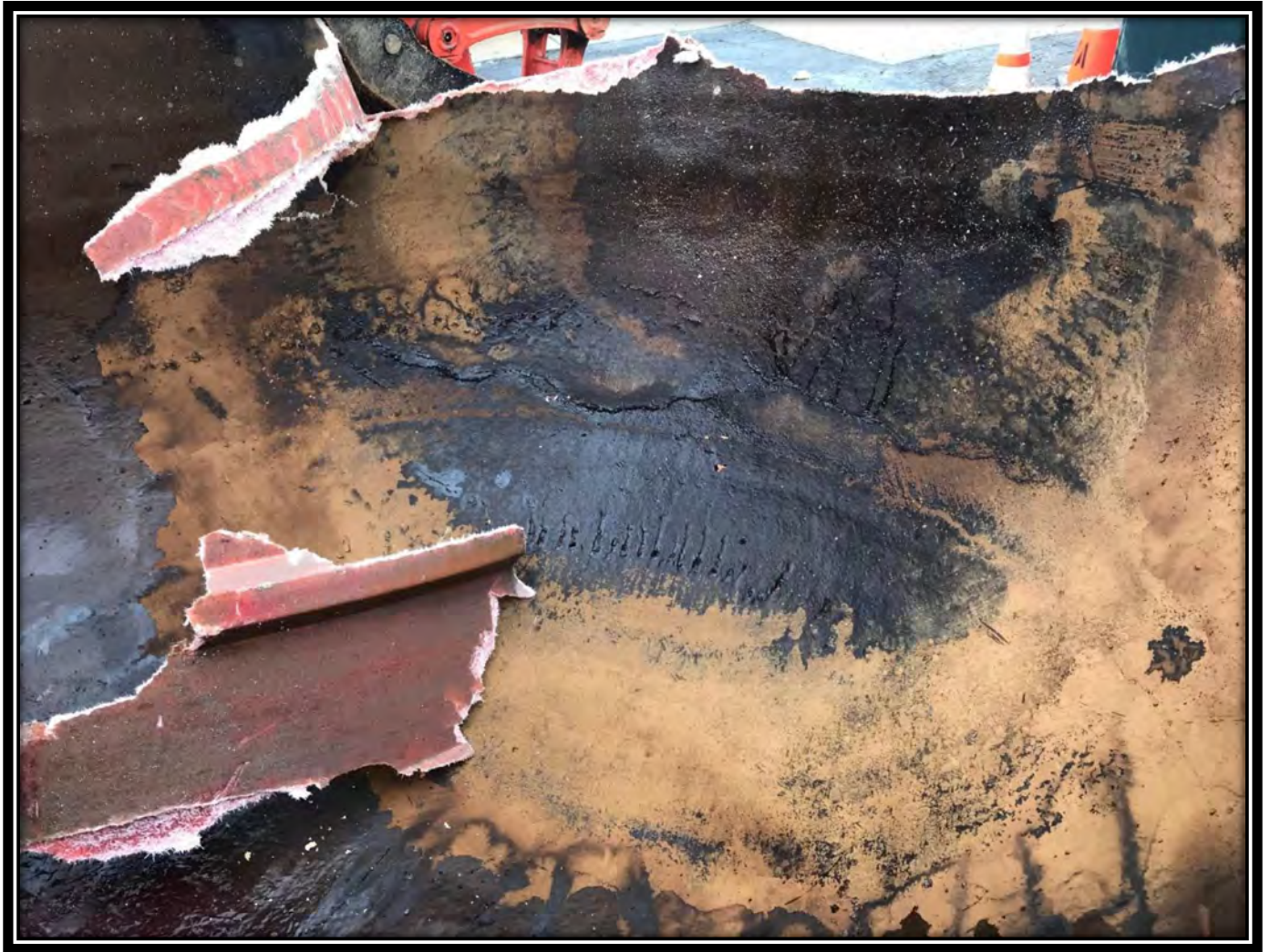
Interior View of Crack in UST 003.
