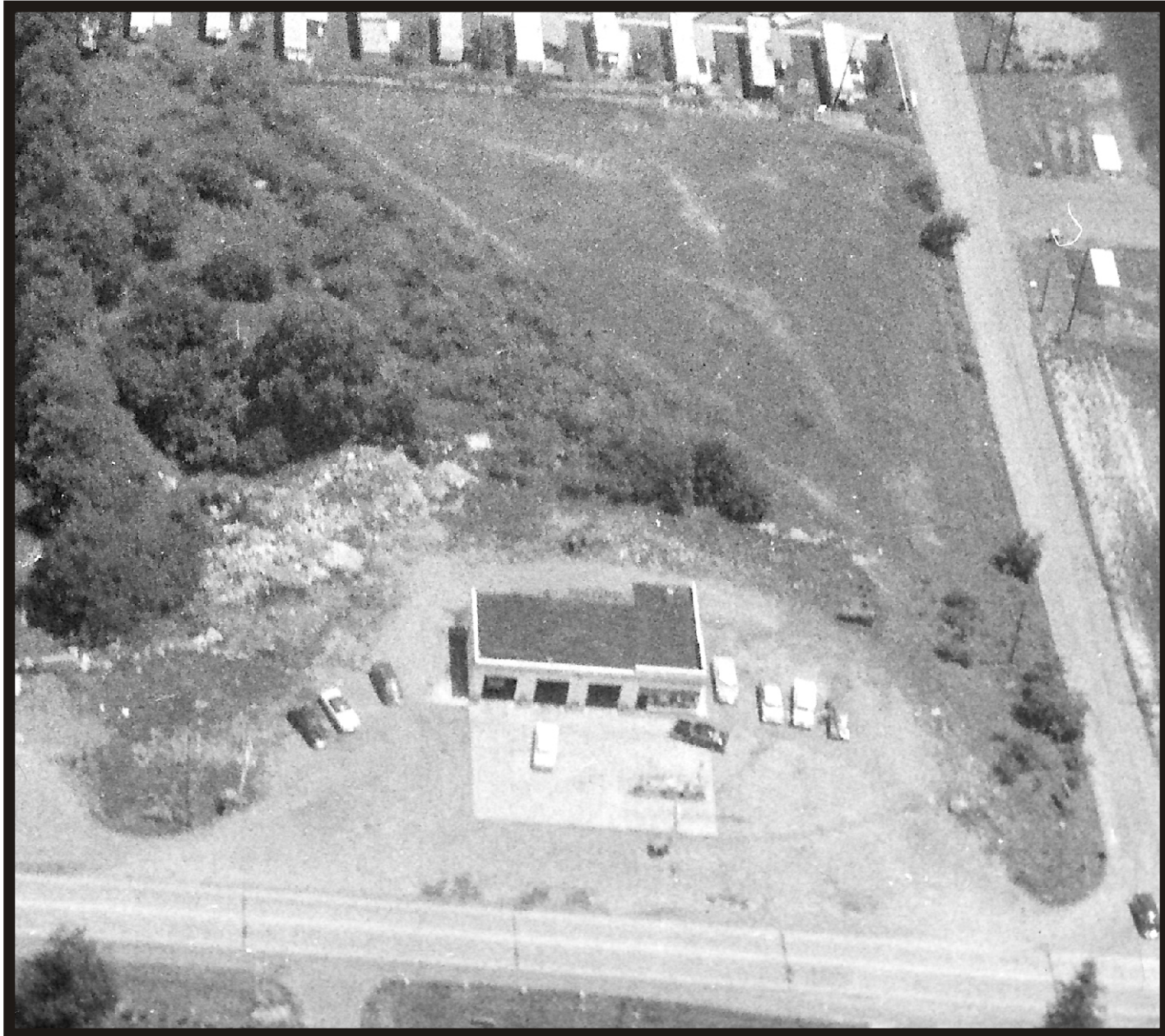
Site Aerial Photography - May 4, 1955 Carlisle Car & Truck Service - Carlisle, Pennsylvania
