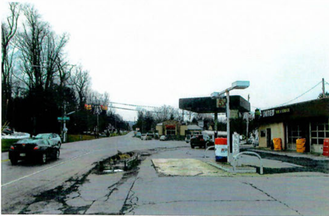
2.0 View along Chestnut Street to the Southwest.
