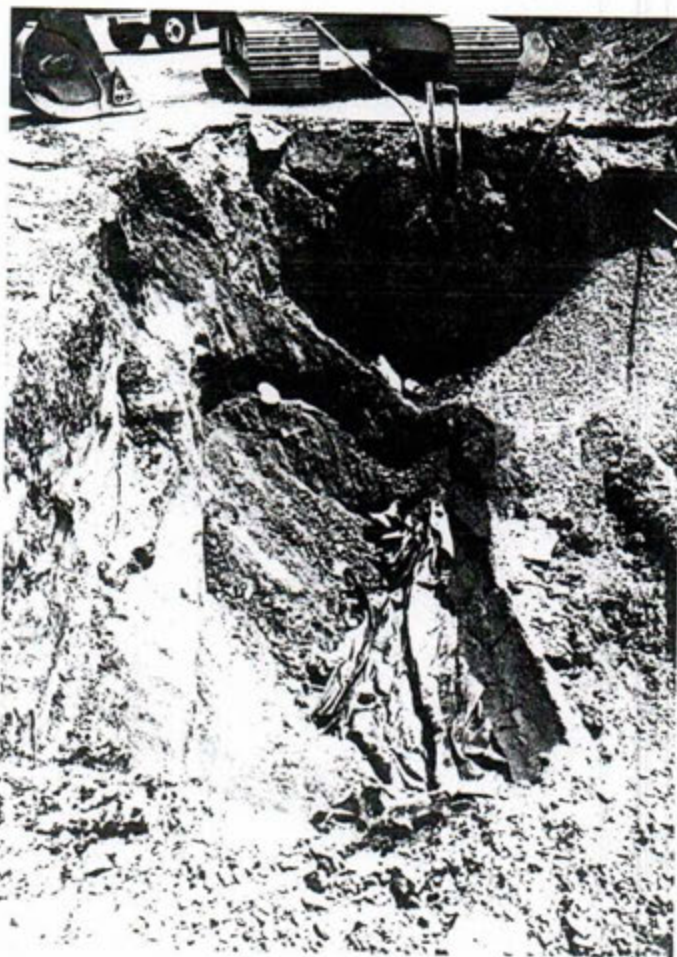
Below: Excavation after 6,000 tank removed
