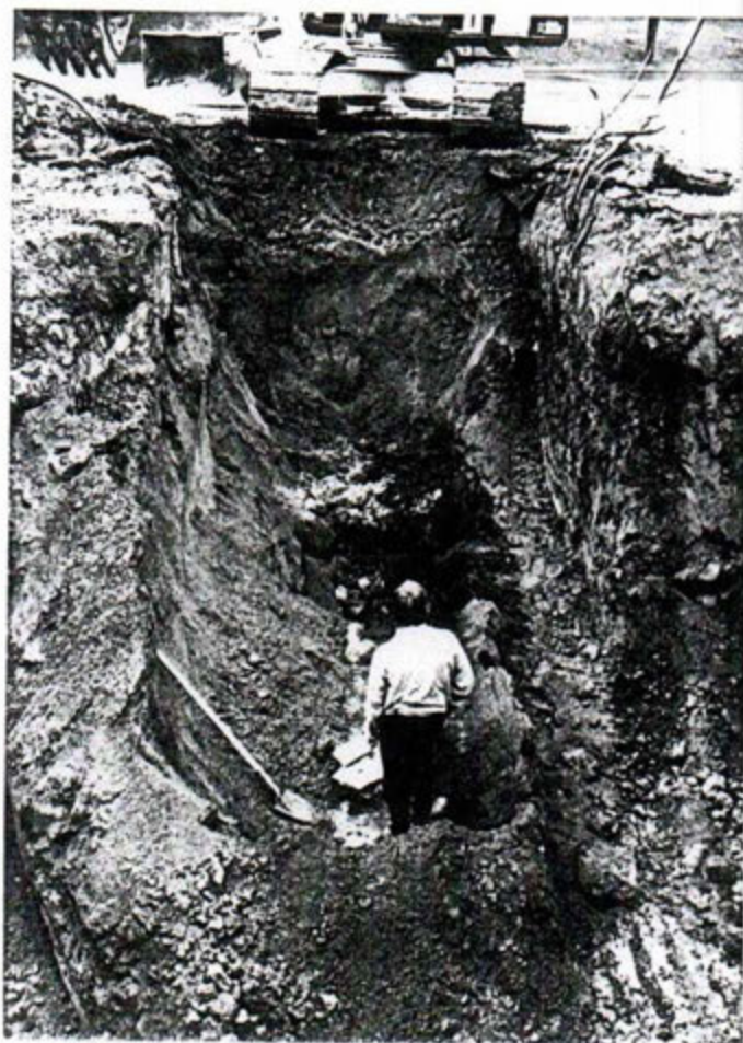
Below: Excavation after 10,000 tank removed
