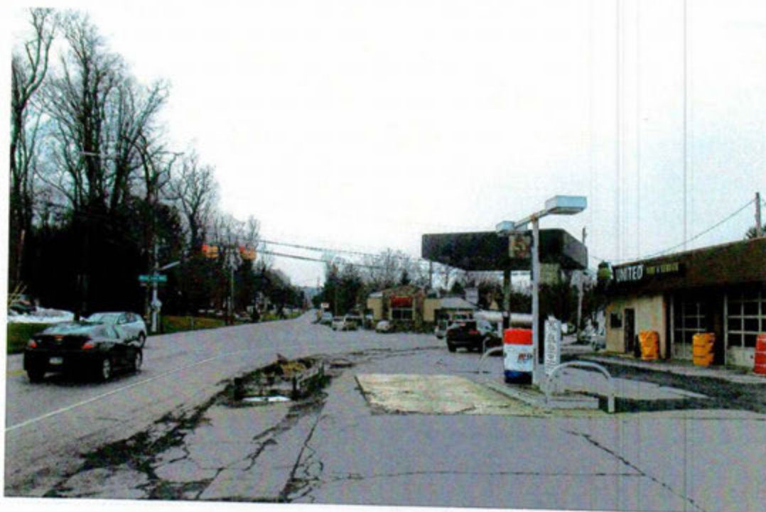
2.0 View along Chestnut Street to the Southwest.
