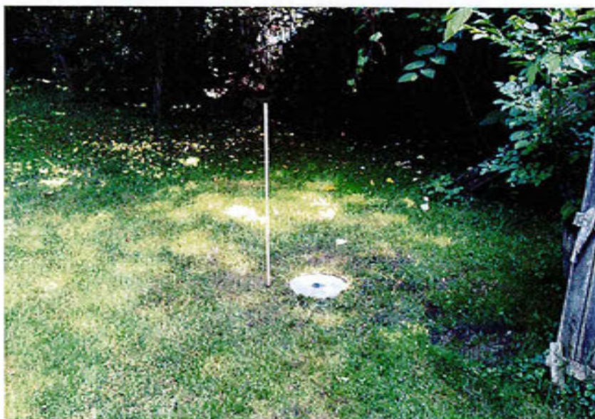
Completed Monitoring Well #18 on Dzikowski
