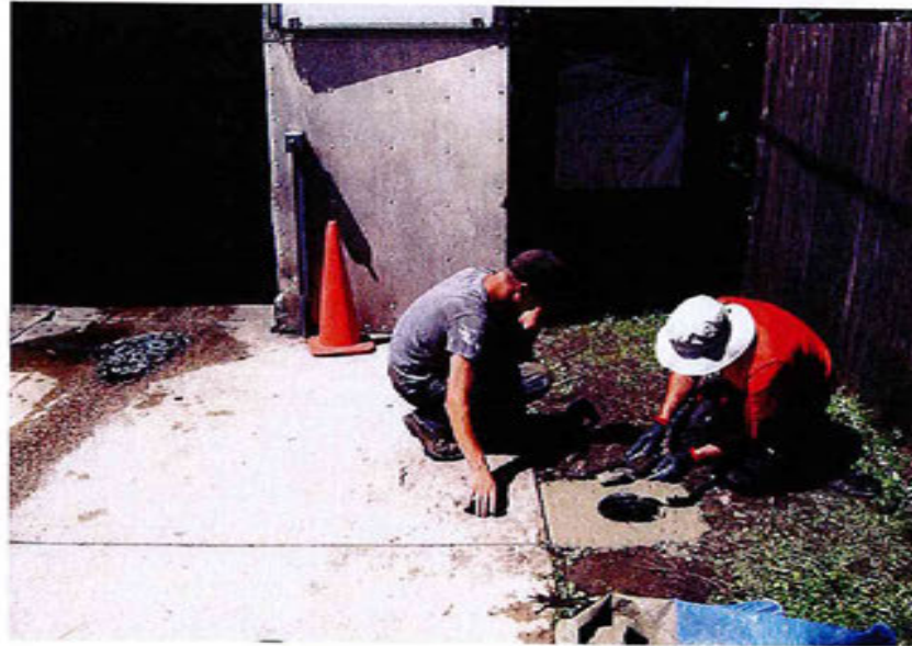
Finishing Cement Around MW #19 on Leo's Site
