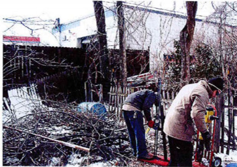
Setting-Up to Advance Off-Site MW #21 on Parker Property
