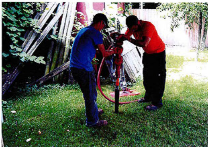
Advancing Off-Site Monitoring Well #18 on Dzikowski
