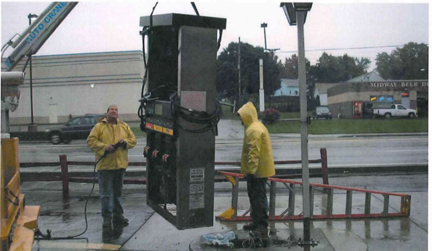
Removing Gas Dispenser
