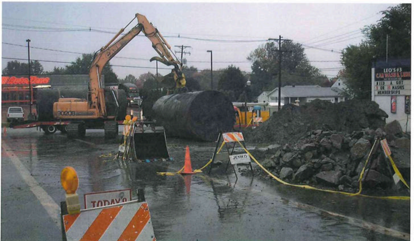
Removing Tanks From Leo's Car Wash
