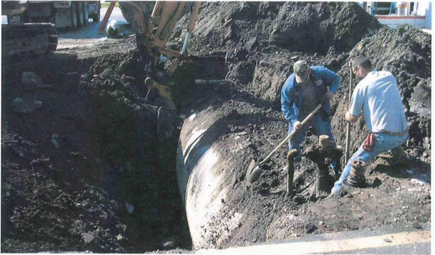
Cleaning Dirt Off of Tank Prior to Removal
