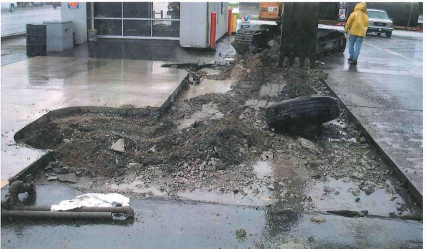
Removing Fill Above Piping
