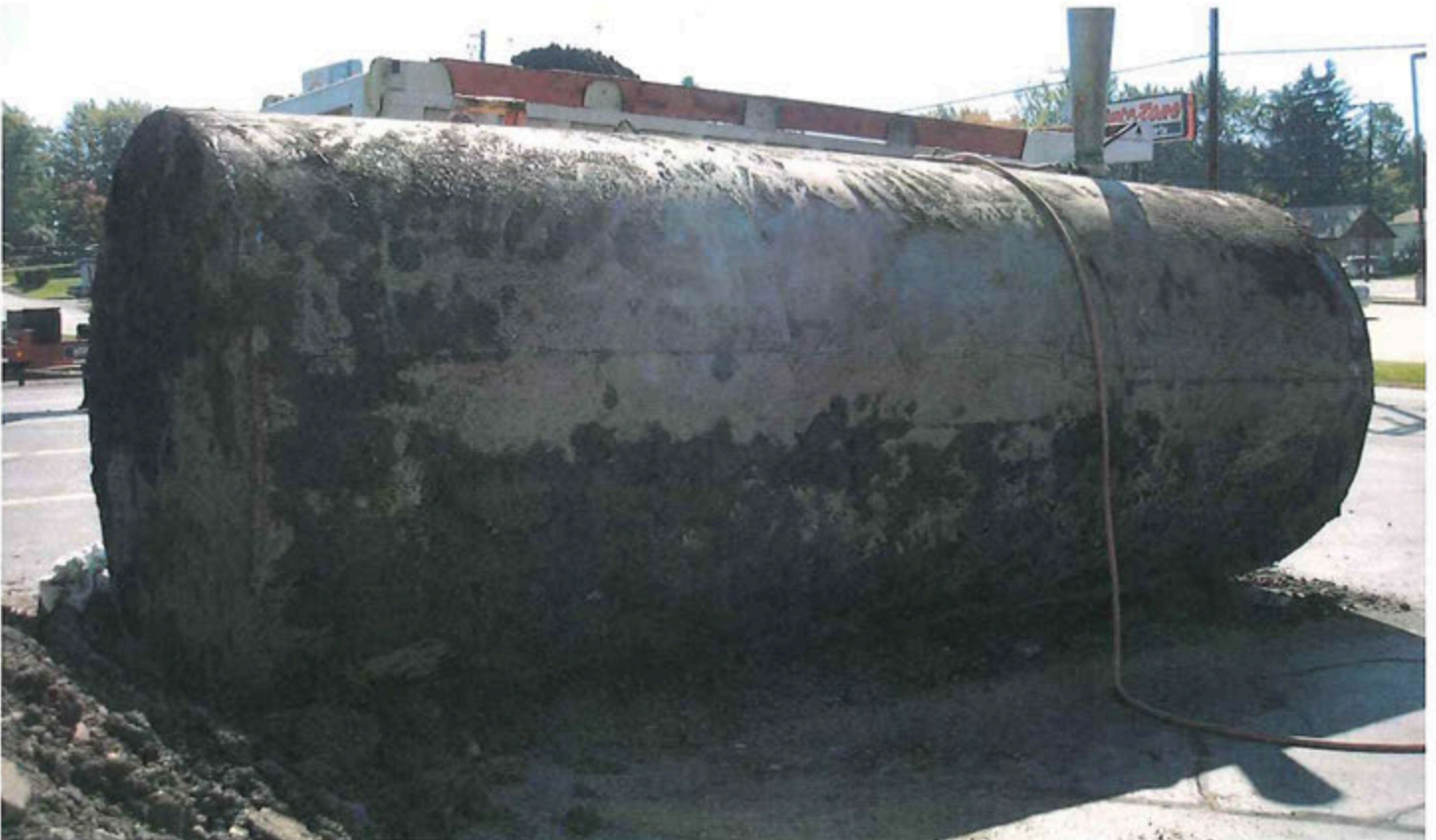
UST In Relatively Good Condition
