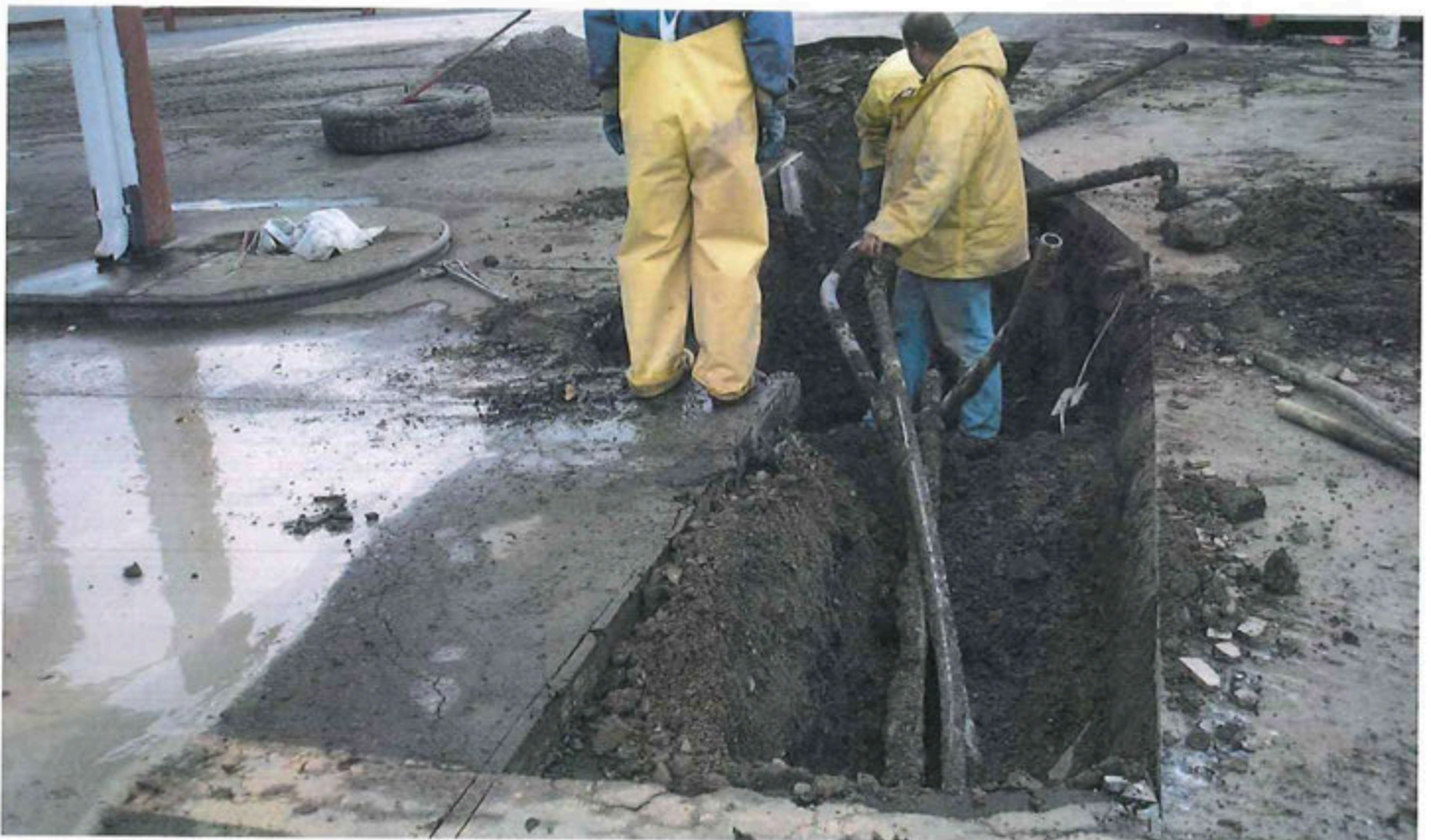
Removing Delivery Line Piping
