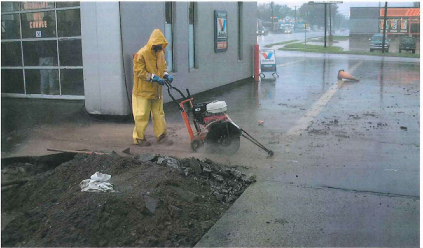
Saw Cutting Prior to Uncovering Piping
