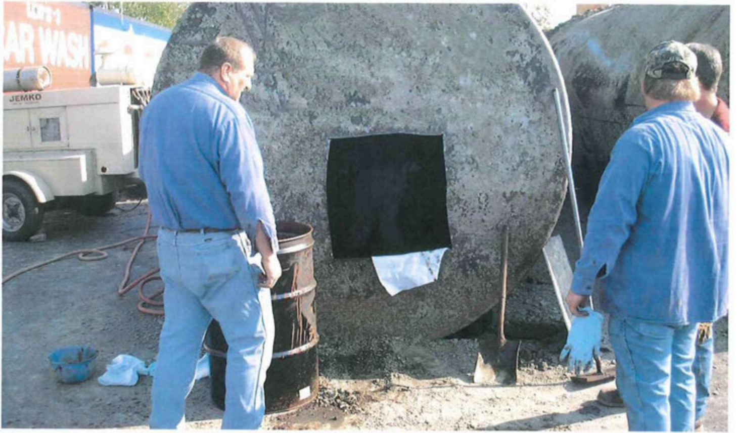
Cleaning of Tanks
