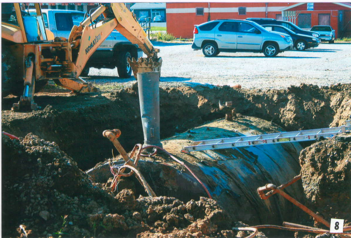
Photograph #6 – Vapor removal from tanks
