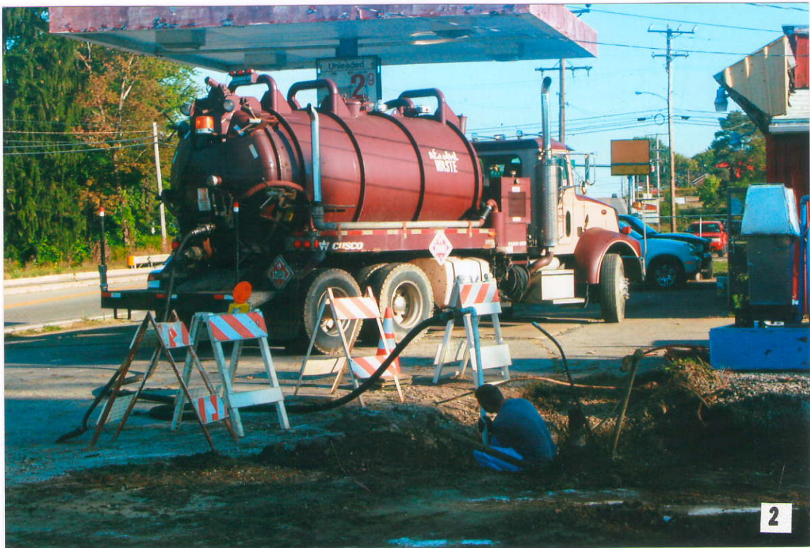
Photograph #1 – Removal of product from tanks
