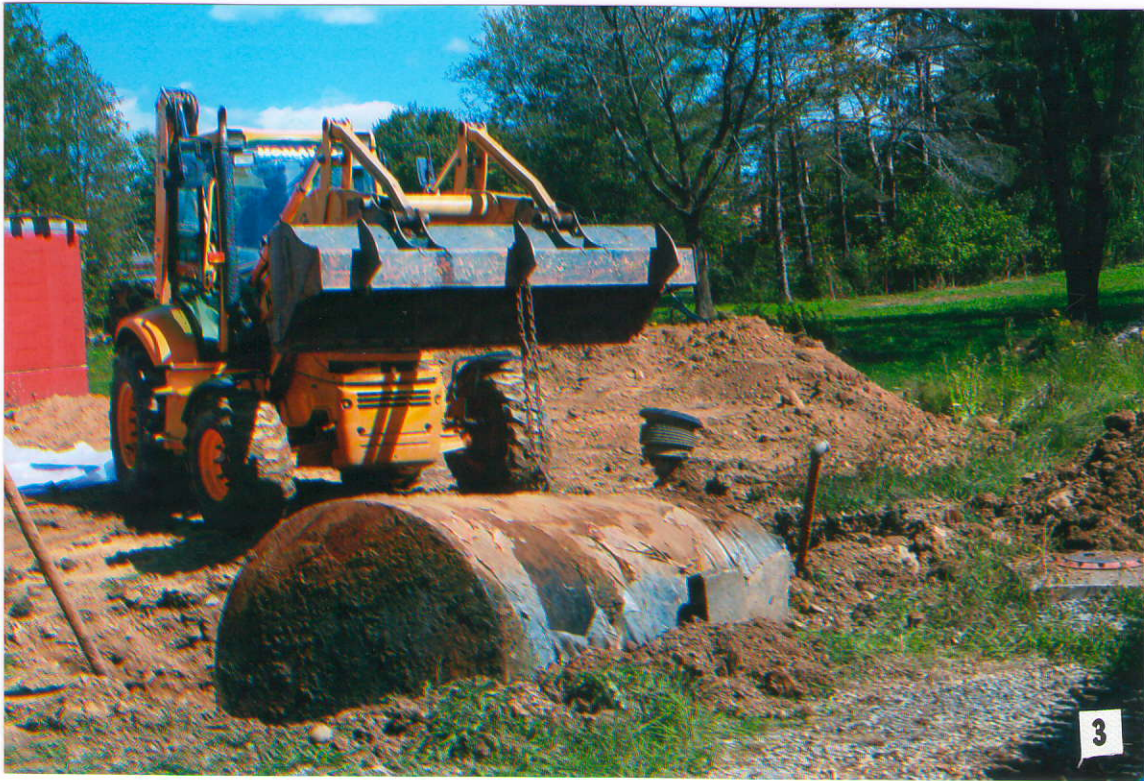
Photograph #3 – Removal of Tank #005 (1000 gallon kerosene)
