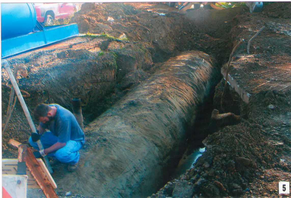
Photograph #7 – Removal of Tank #001 (6000 gallon gasoline)
