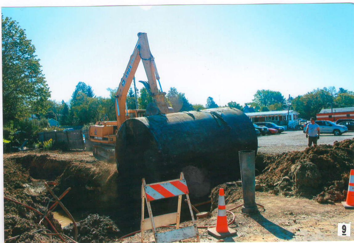
Photograph #8 – Removal of Tank #003 (10,000 gallon gasoline)
