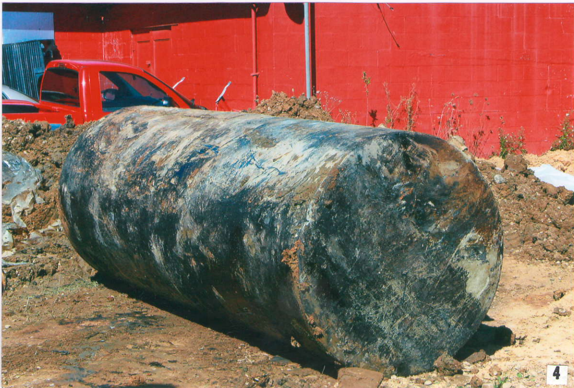
Photograph #4 – Removal of Tank #004 (2,000 gallon diesel)
