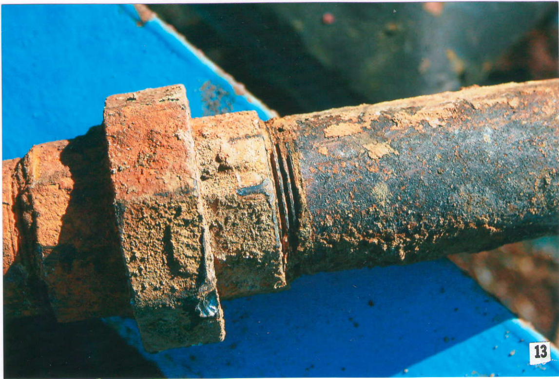
Photograph #11 – Leaking fitting on Tank #003
