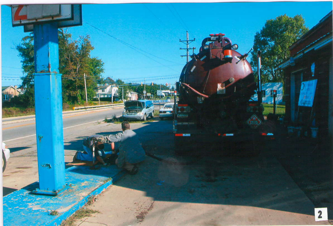
Photograph #2 – Removal product from lines
